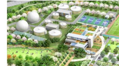
Administrative Complex City Water Quality Restoration Center A-2, 3 Beneficiary: Sejong City Capacity: 60,000m 3 /day
