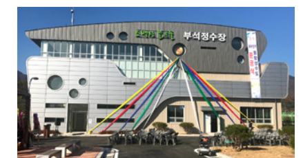
Yeongju City Buseok Water Purification Plant Beneficiary: Yeongju Capacity: 2,100m 3 /day
