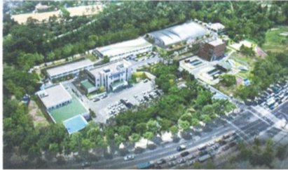
Gongsan Drinking Water Treatment Plant in Daegu Client ----- Daegu City Capacity ----- 40,000m 3 /day
