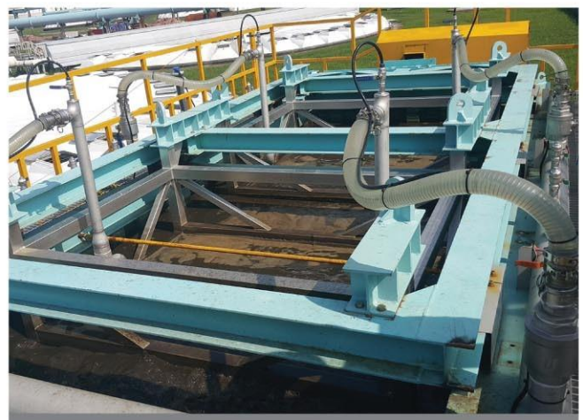
Kolon Membrane is applied for Doosan LENA (Low Energy No Aeration) MBR
