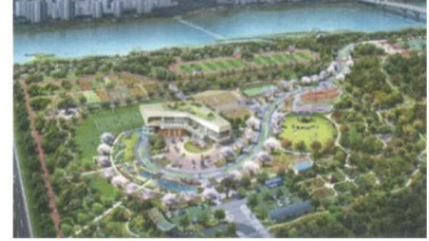
Sejong City Sewage Treatment Plant Client ----- Sejong City Capacity ----- 80,000m 3 /day
