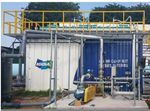
Kolon Membrane is applied for Doosan LENA (Low Energy No Aeration) MBR
