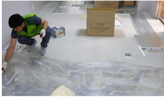
Panel installation following bond application (1)
