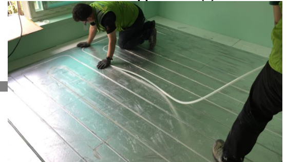
Pipe installation
