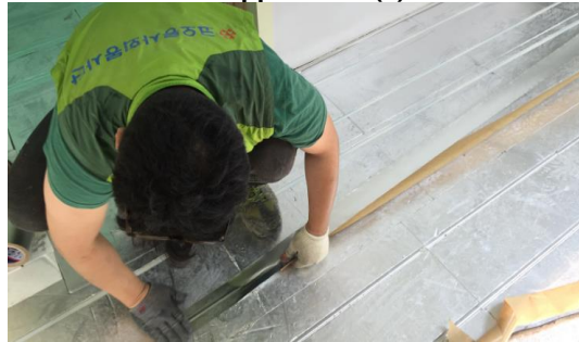
Application of aluminum tape
