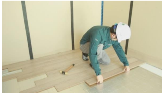
Installation of laminate flooring
